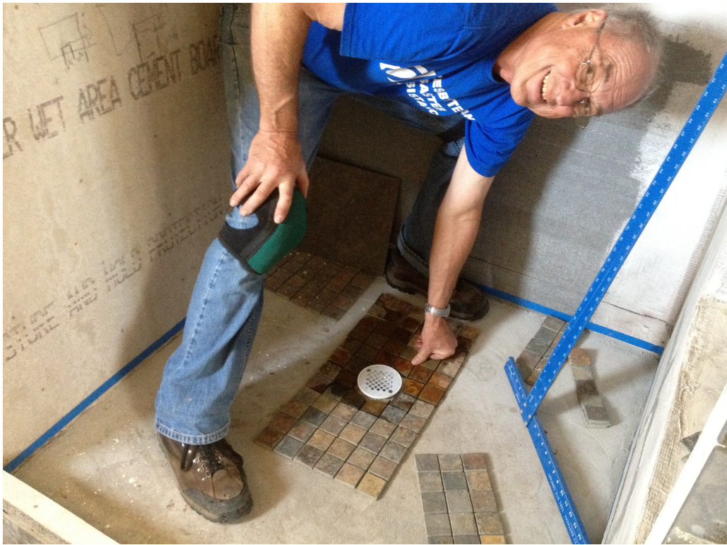
Getting a start on laying the floor tile
