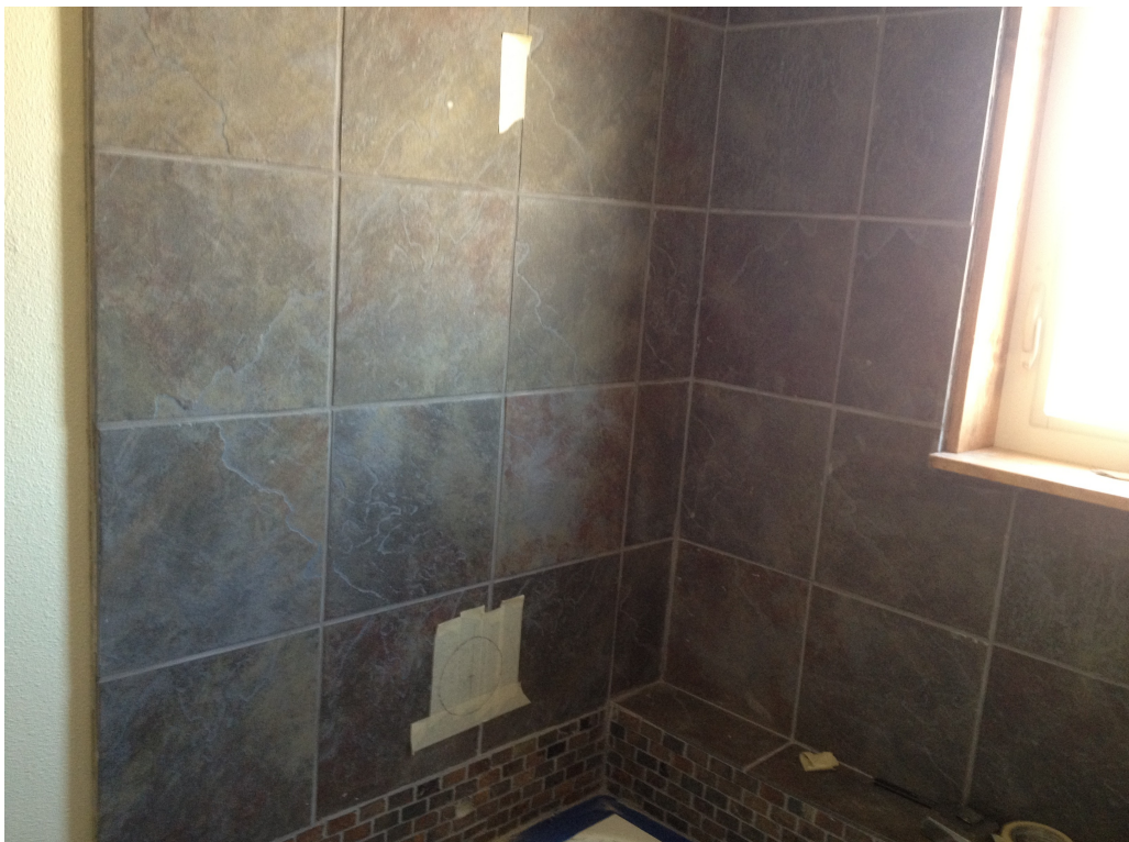
Marking where the holes are to be cut for the plumbing
